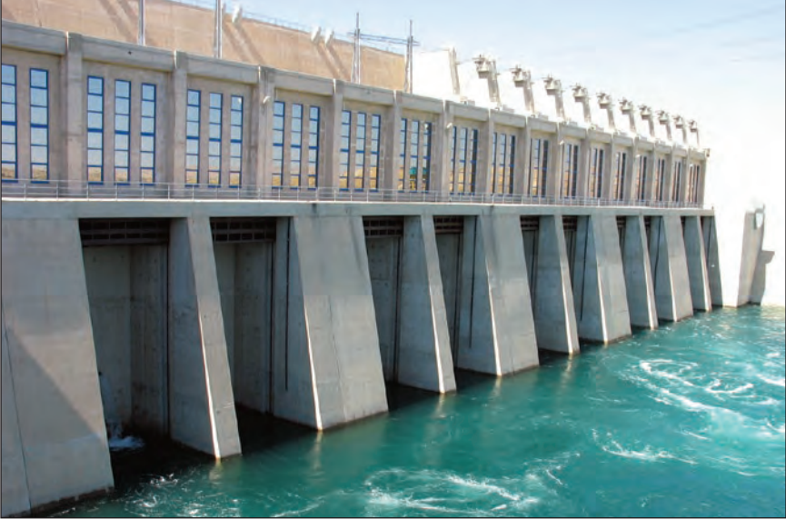
Figure 5.2. Karkamis Dam on the Euphrates River, southern Turkey
