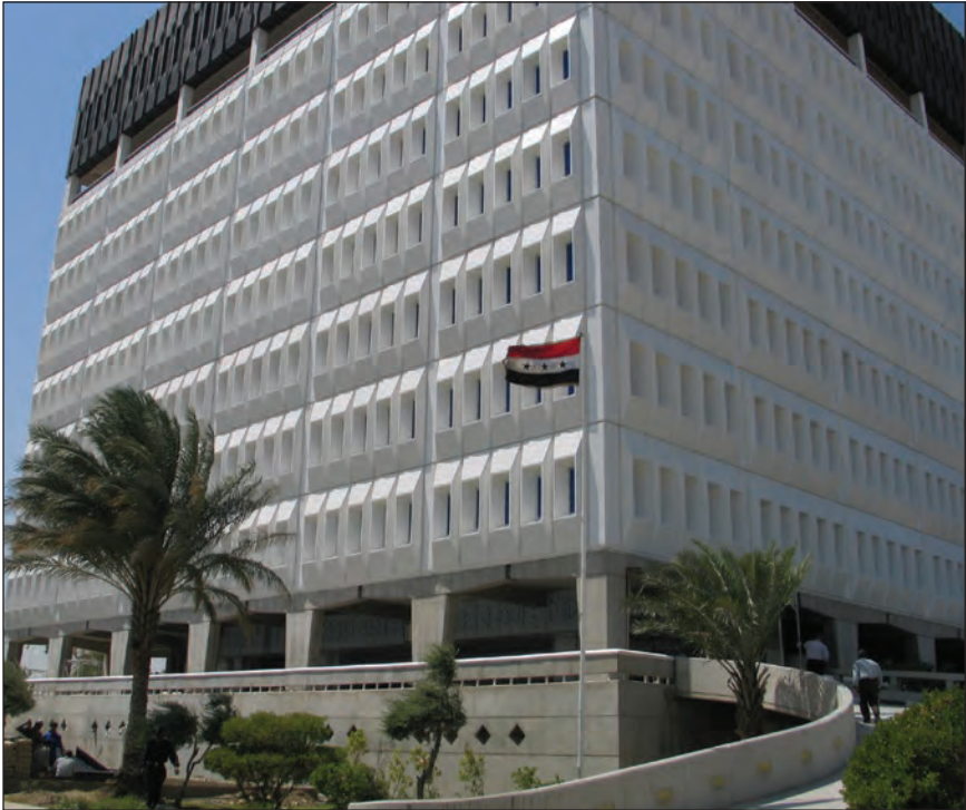
Figure 6.2. Iraqi Ministry of Water Resources building, Baghdad
